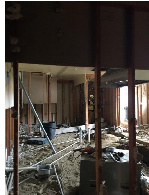
NEW PLUMBING IN KITCHEN
