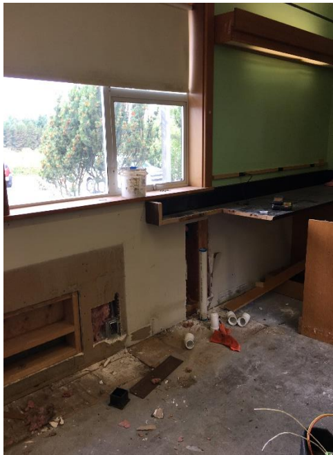
NEW ELECTRIC AND PLUMBING IN THE SCIENCE LAB
