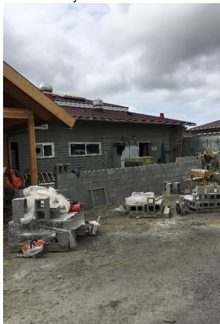
NEW WALLS AT SERVICE YARD/KITCHEN
