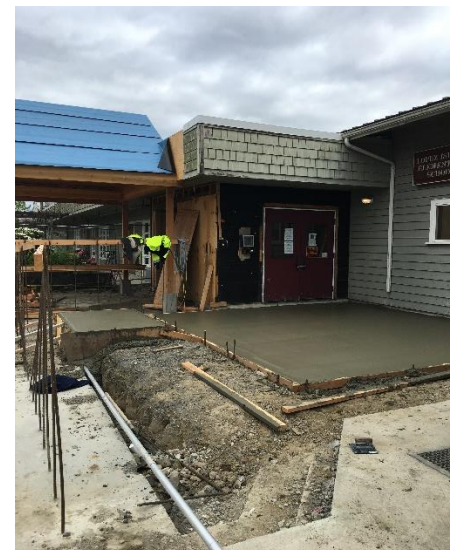
ENTRY ROOF DRIED IN AND NEW CONCRETE FOR NEW FREEZER
