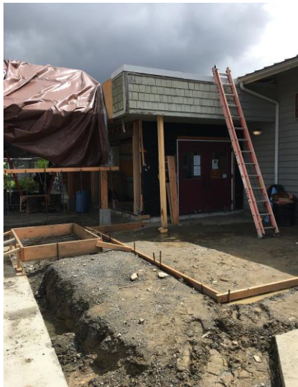
ONGOING FORM WORK FOR KITCHEN
