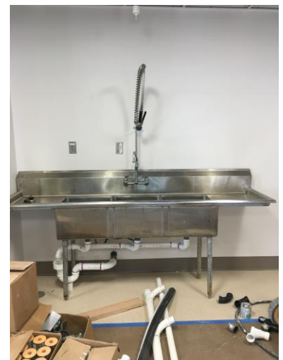
3 COMPARTMENT SINK FOR TEMPORARY KITCHEN
