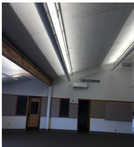
NEW LIGHTING AND PAINT IN MUSIC RM
