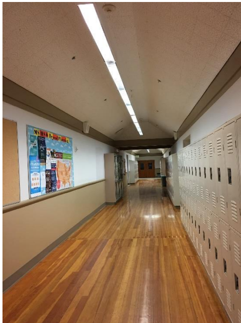
NEW PAINT AND BASE IN SECONDARY HALLWAY
