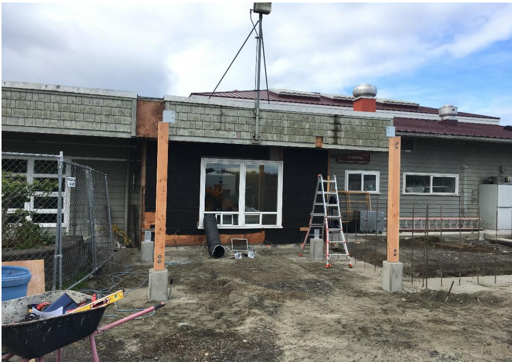
NEW FOUNDATIONS AND FRAMING AT ELEMENTARY ENTRANCE
