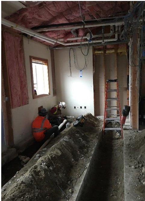
INSTALLING UNDERGROUND PLUMBING IN NEW CULINARY
