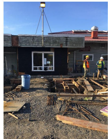
NEW FOUNDATIONS FOR ES ENTRY
