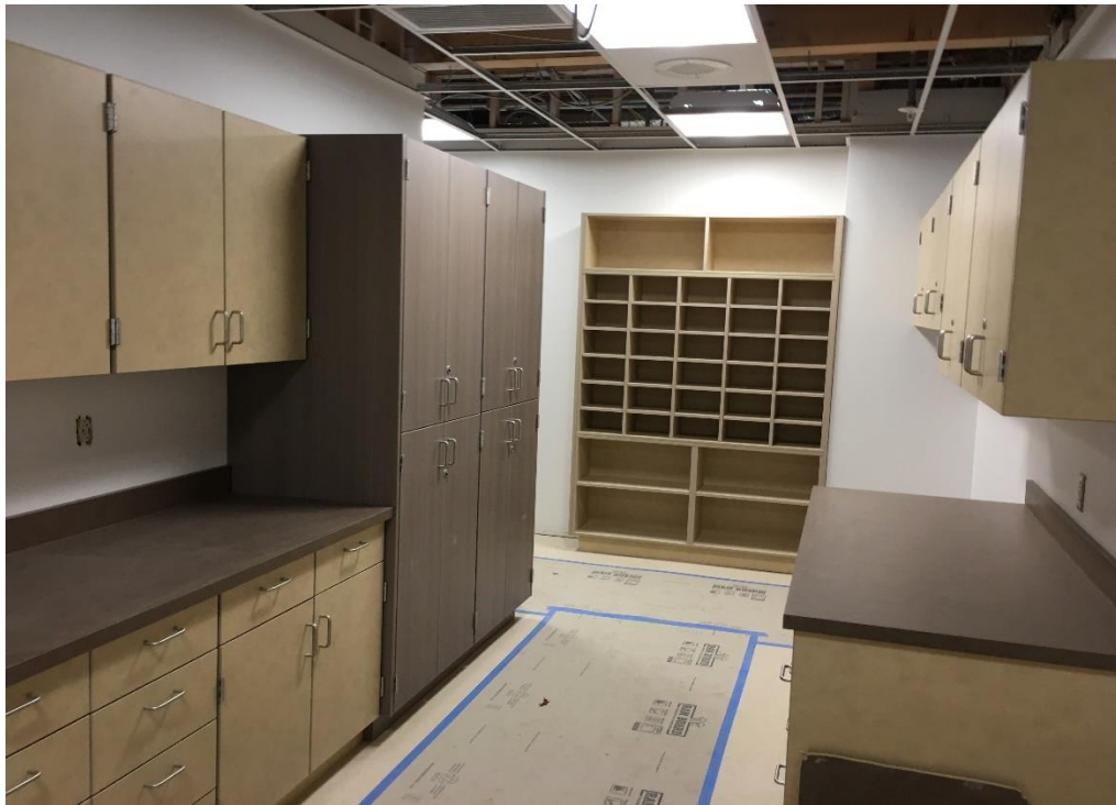
NEW CASEWORK IN ES OFFICES
