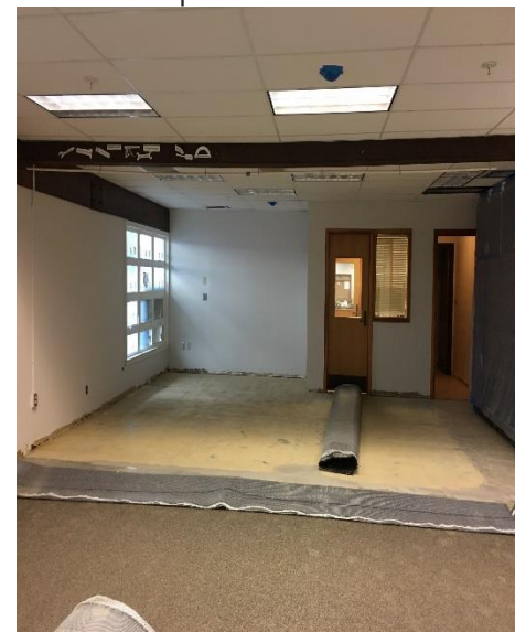
NEW FLOORING IN CLASSROOMS
