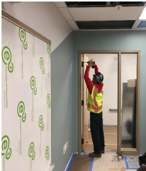
NEW DOORS AND HARDWARE IN ES OFFICES
