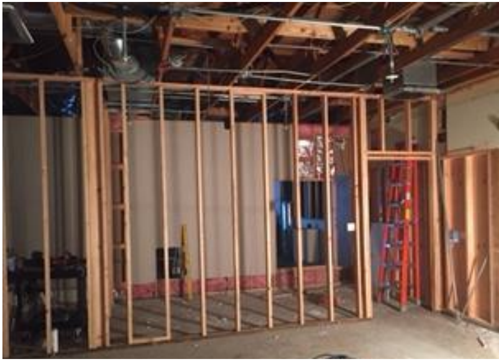
ES CLASSROOMS NEW FRAMING
