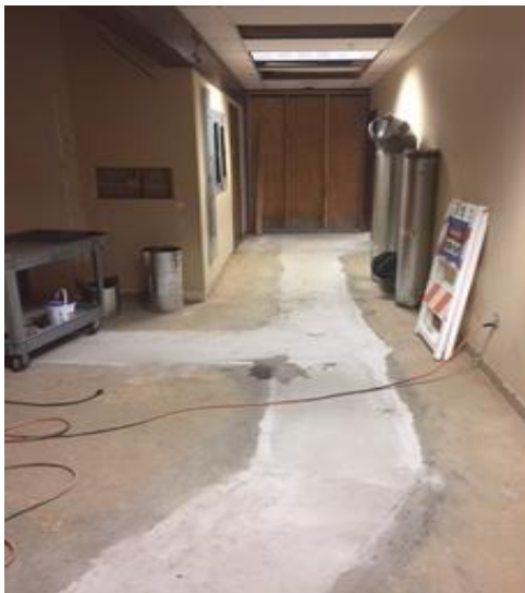
ES CLASSROOMS NEW CONCRETE
