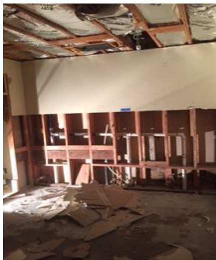
ES RESTROOM DEMOLITION IN PROGRESS
