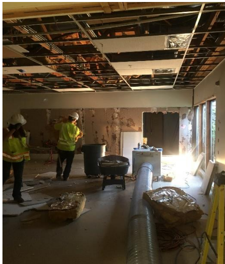
ES8 / POD DEMOLITION IN PROGRESS
