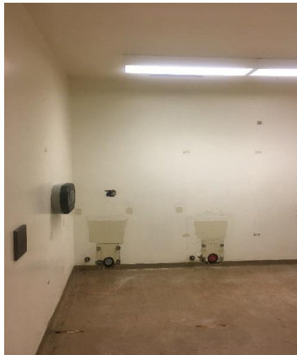
ES BOYS RESTROOM DEMOLITION IN PROGRESS
