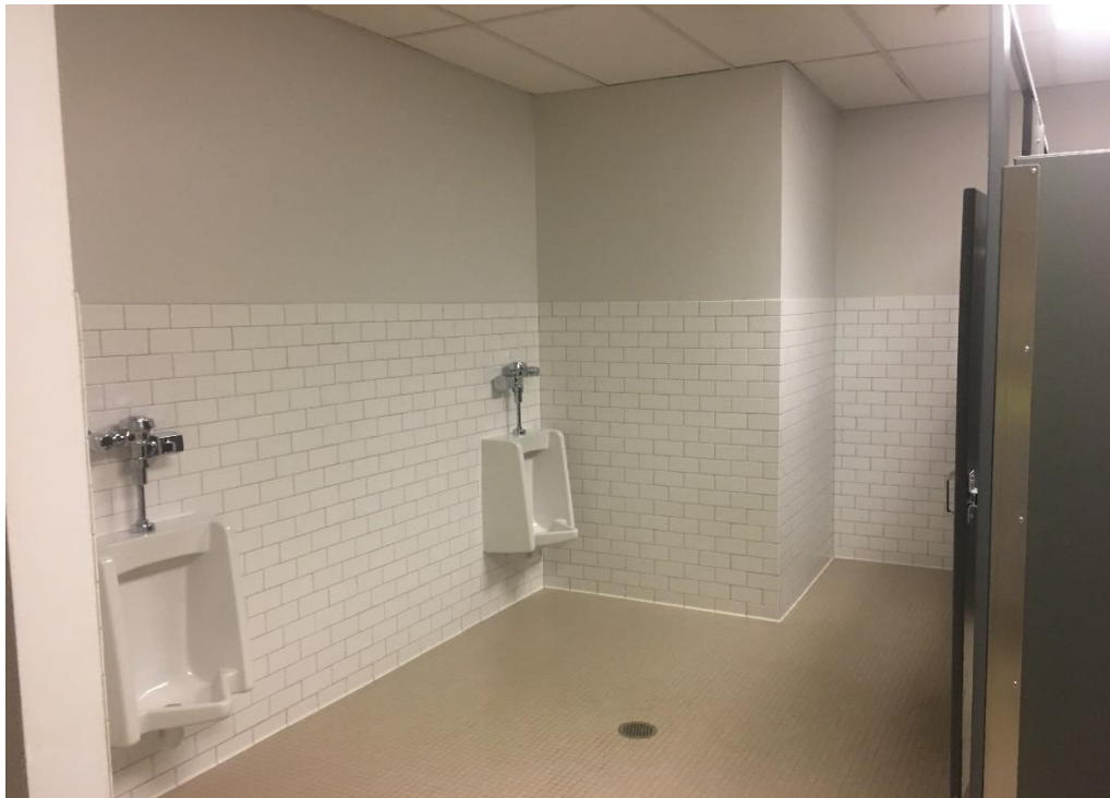
HS / MS BOYS RESTROOM IMPROVED AND READY TO USE
