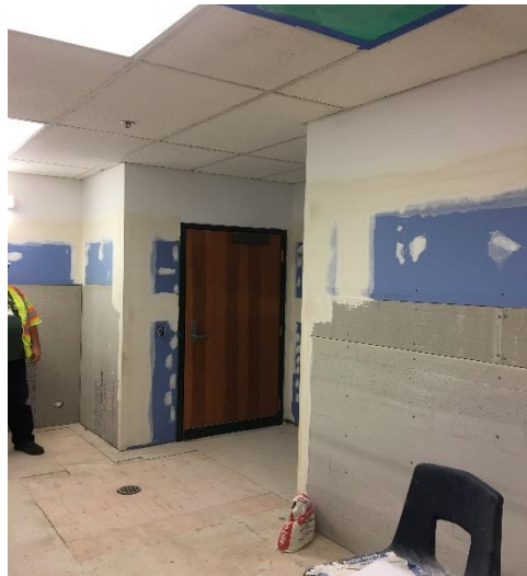
PATCH WALLS FOR CERAMIC TILE
