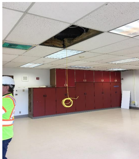
NEW VINYL FLOORING IN CLASSROOMS
