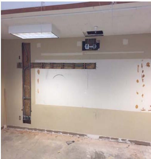
ROUGH IN ELECTRICAL FOR NEW PROJECTORS
