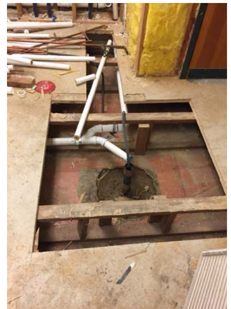
REPAIR FLOORS IN RESTROOMS
