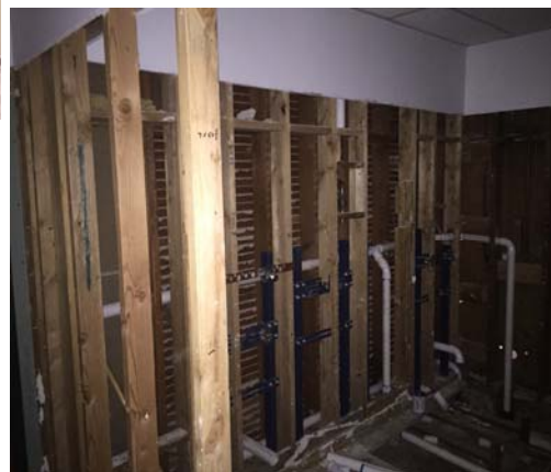
NEW PLUMBING IN RESTROOMS
