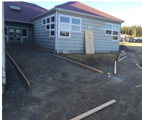
GRADING AND FORMING FOR NEW SIDEWALKS.
