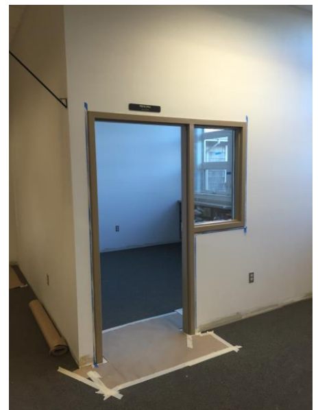
FINISH PAINT AND CARPET IN MS / HS ADMINISTRATION OFFICES.
