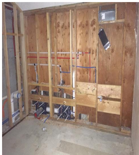
COMPLETED FRAMING AND MEP ROUGH IN AT MS / HS RESTROOMS.
