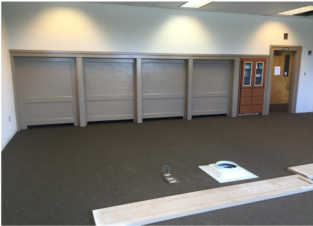
FINISH PAINT AND NEW CARPET IN MS / HS CLASSROOMS.
