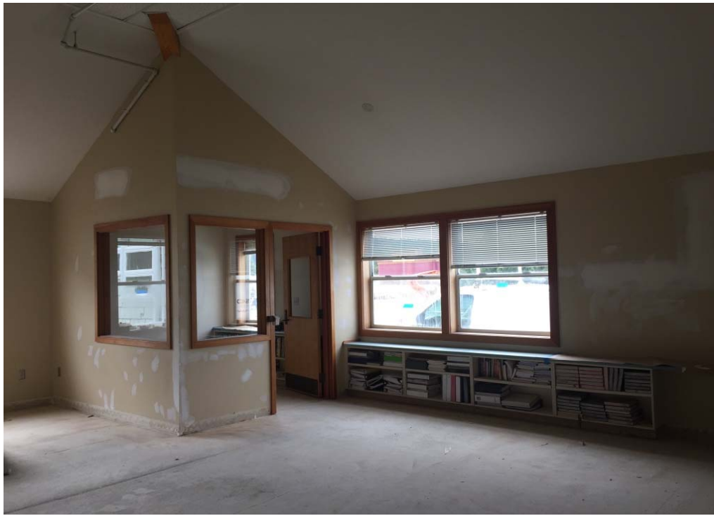
DRYWALL PATCH AND REPAIR IN MS / HS CLASSROOMS.
