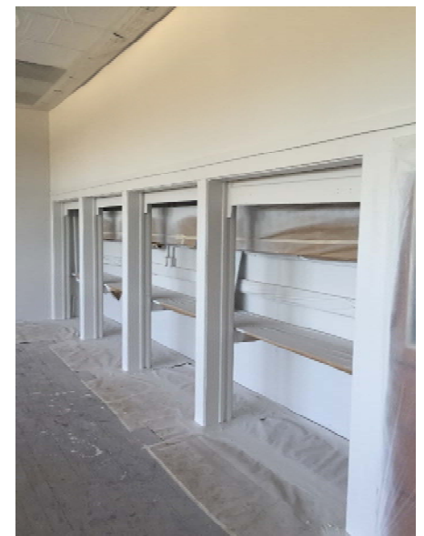
MS / HS CLASSROOM DRYWALL PATCHING AND PAINTING.
