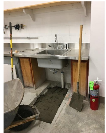
NEW SINK AND SS COUNTER IN SHOP
