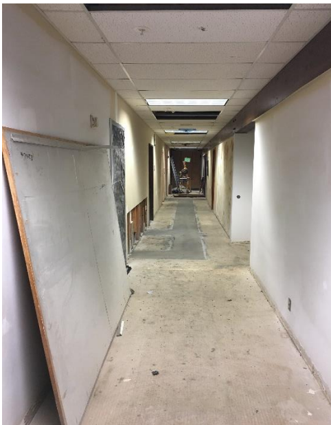
INFILLED FLOOR OVER NEW SANITARY IN ES
