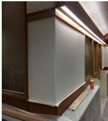
NEW PAINT IN LIBRARY
